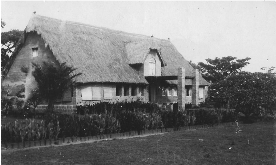
"House designed and built by EWTM of ironstone blocks. Ironstone when first exposed to air is quite soft and can be trimmed with an axe." (Tom on back)
